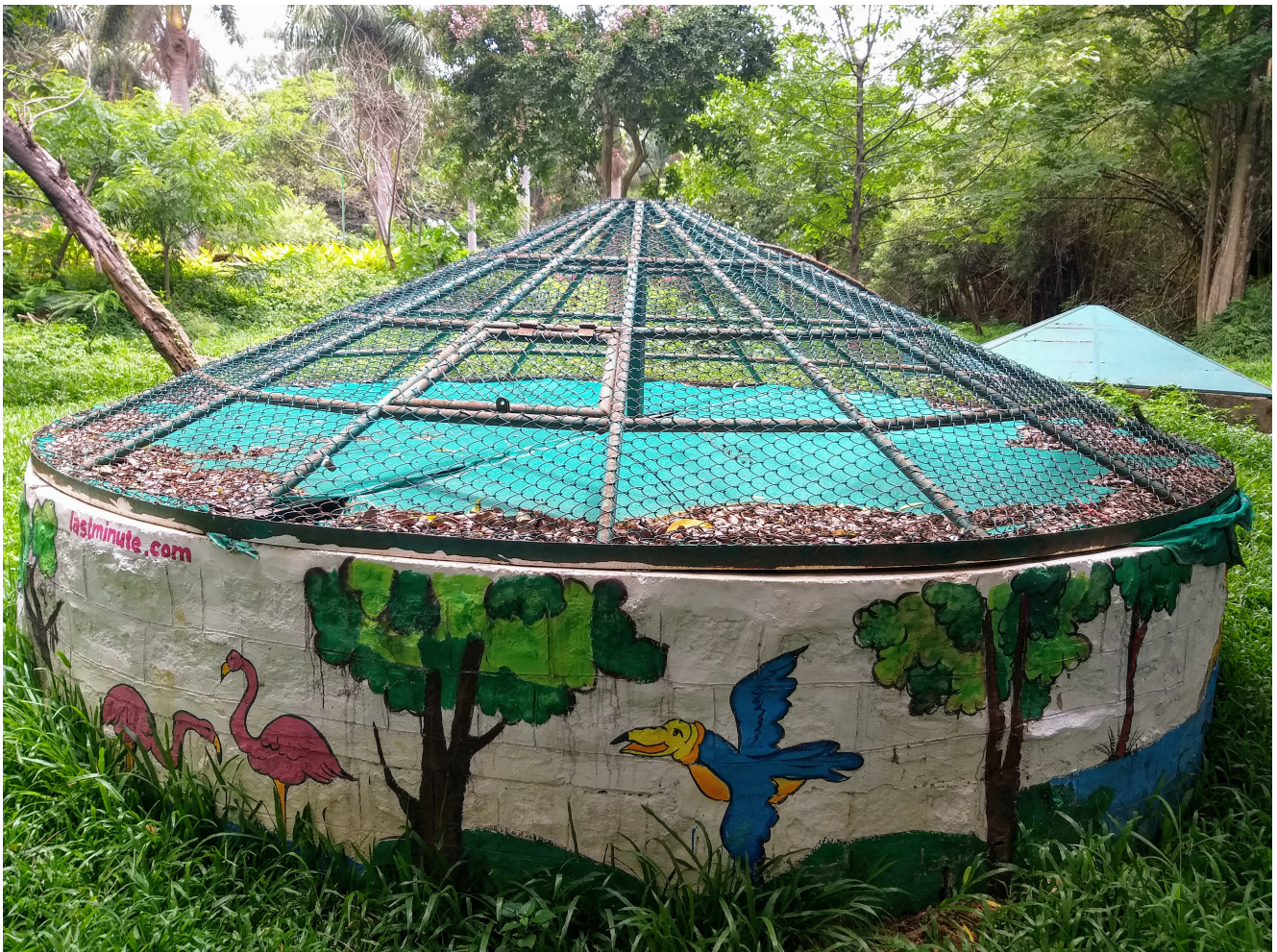
Open recharge well in the city Image courtesy of Mr. Vishwanath Srikantaiah
