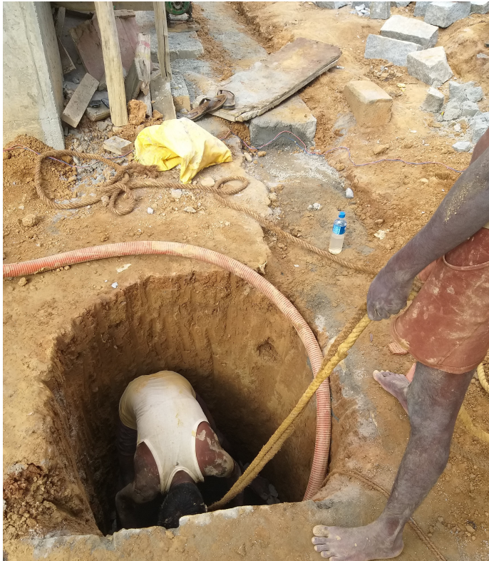
Mannu Vaddars digging a recharge well Image courtesy of Mr. Vishwanath Srikantaiah
