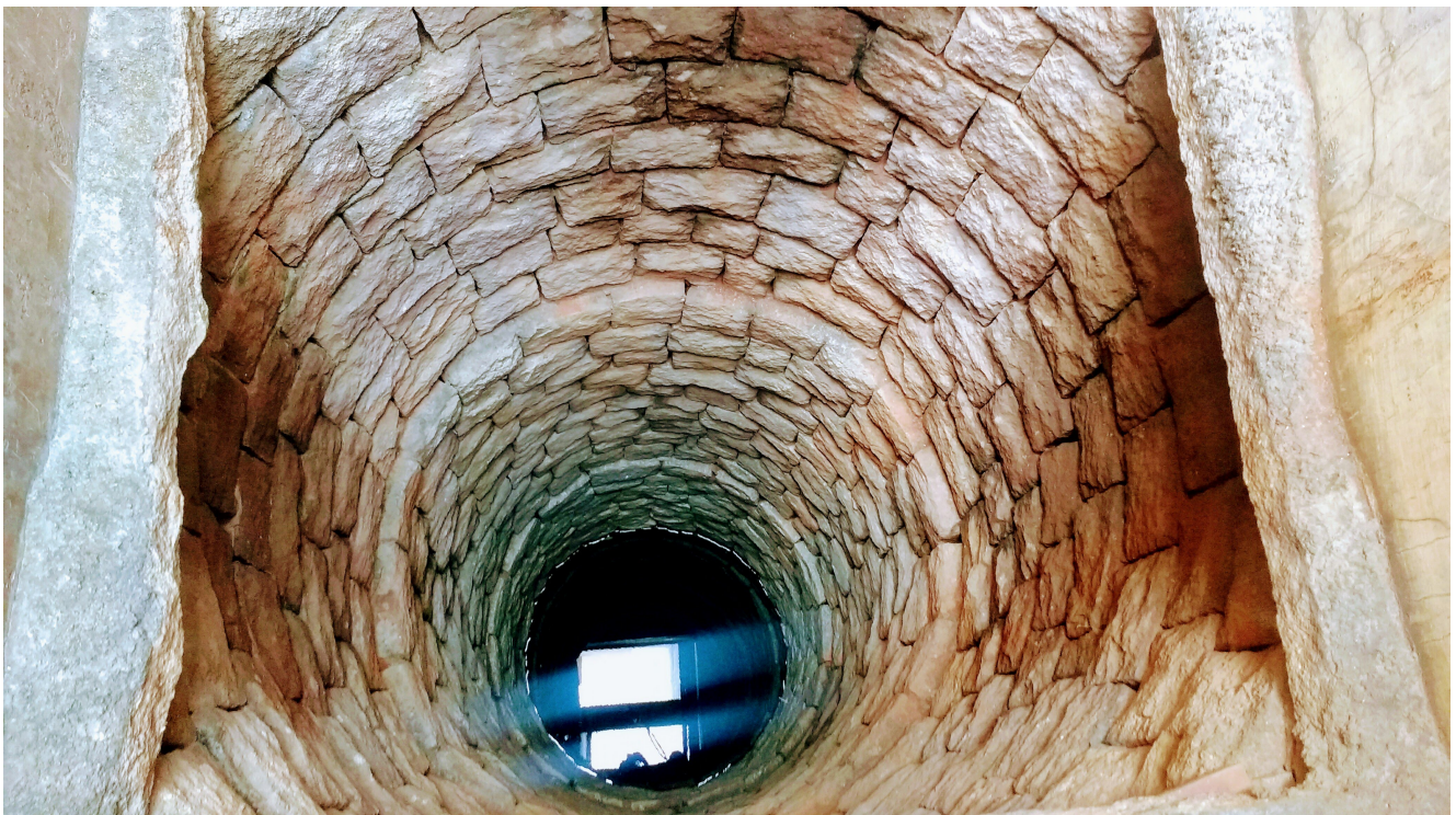
Old stone-lined well recharged with rainwater Image courtesy of Mr. Vishwanath Srikantaiah
