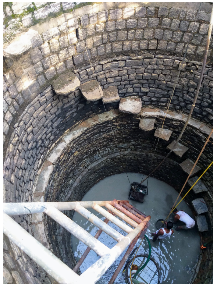
Mannu Vaddars cleaning and desilting a recharge well Image courtesy of Mr. Vishwanath Srikantiah
