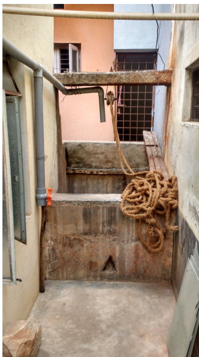
Rooftop rainwater recharging a well Image courtesy of Mr. Vishwanath Srikantaiah
