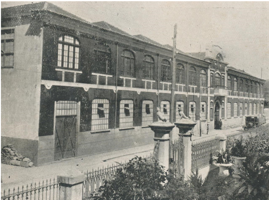
Figure 1 Confiança Factory in 1928. Source: Jornal Arquitectos
