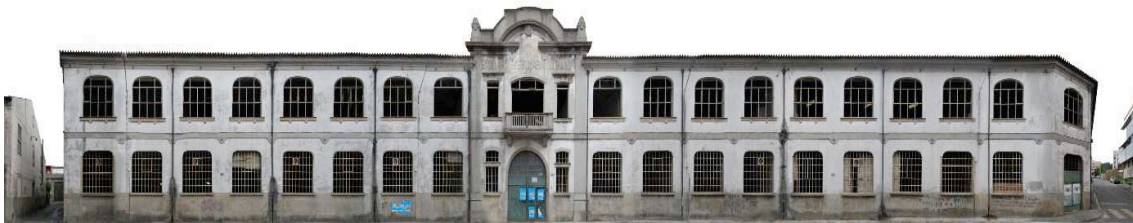
Figure 2 Building of Confiança, today. Source: (Guimarães, 2014)
